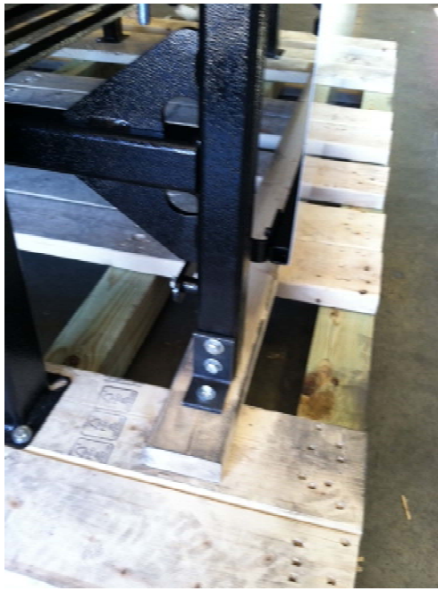
LOWER ANGLE BRACKET BRACING
