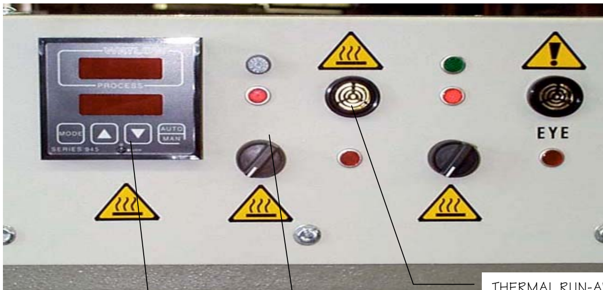
TEMPERATURE CONTROL CONTROL POWER ON/OFF THERMAL RUN-AWAY ALARM
