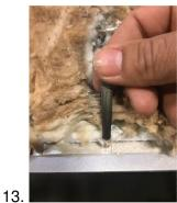
Slide the black sleeve tube over the heat element wire & cut the black tubing so only <sup>1</sup>/<sub>4</sub>" of the wire is showing. Then strip the end of the wire <sup>1</sup>/<sub>4</sub>".
