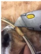
Use the utility knife to carefully cut any white cloth tape that is used to keep wires together. Then remove the cut tape itself.
